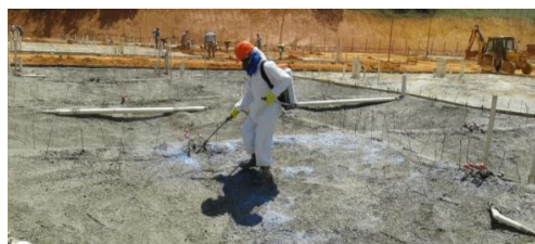
Fig. 12 Chemical curing after concreting the modules
