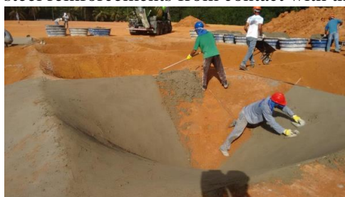
Fig. 6 Applying the mortar layer for regularization
