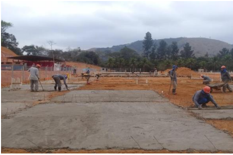
Fig. 14 Applying of the mortar layer to regularise the embankment
