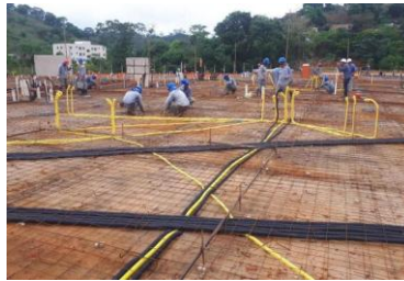
Fig. 15 Assembly steel reinforcement of slab and building installations
