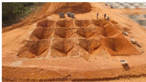
Fig. 4 Excavation of the membrane modules
