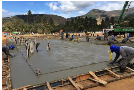
Fig. 16 Slab concreting
