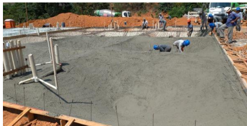
Fig. 11 Concreting the modules
