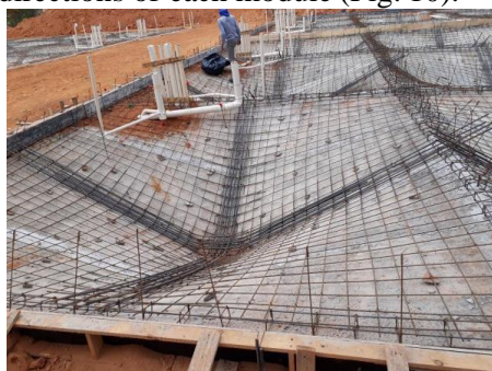
Fig. 10 Placing the steel reinforcement in the modules
