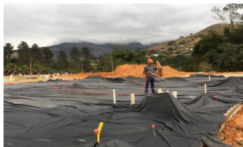
Fig. 17 Concrete curing after slab concreting
