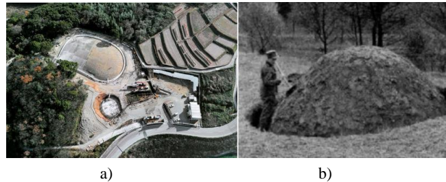
Fig. 1 a) Earth formwork for the Teshima Art, b) Isler's freely shaped hill method [12]
