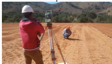
Fig. 3 Localisation of the modules with the help of topography
