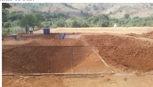
Fig. 5 Regularisation of modules using the template
